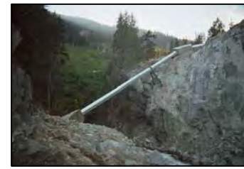
Miller Creek - Pipe Bridge
