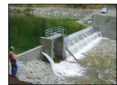
McNair Creek - Intake and Headpond
