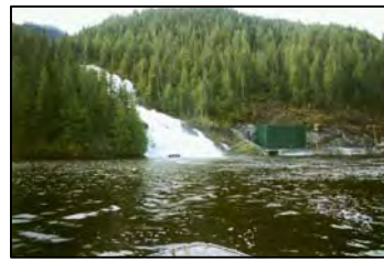
Brown Lake - Powerhouse
