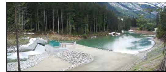
Rutherford Creek - Rubber Weir Intake
